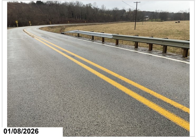
Beginning left approach railing replaced.
