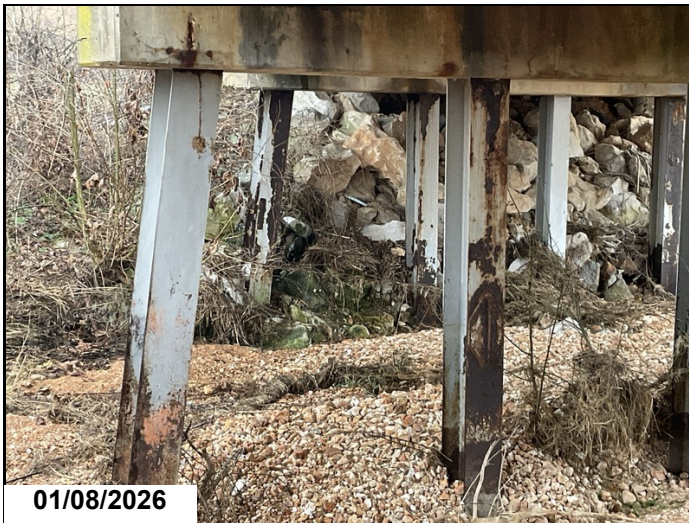
Rip rap has been replaced at abutment #1.
