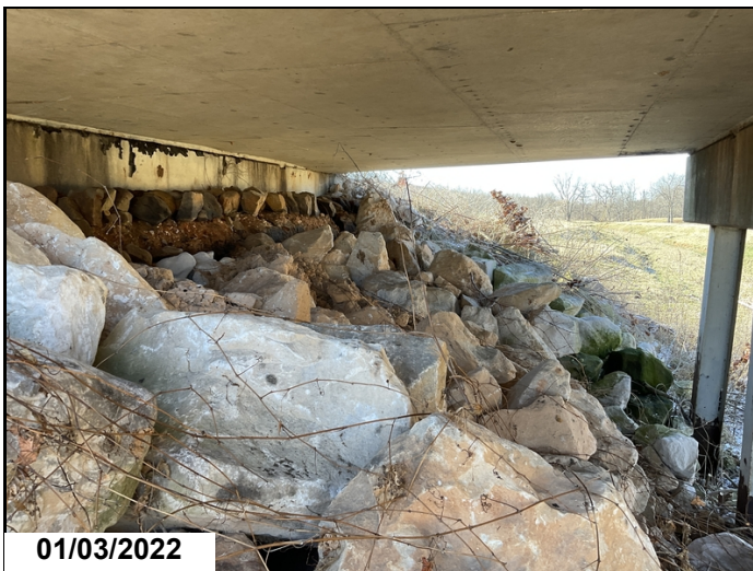
Embankment at abutment #1 settlement.
